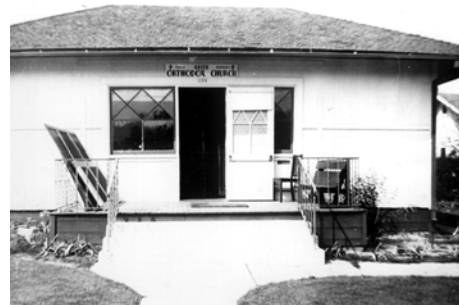
First building used as a Church sanctuary
